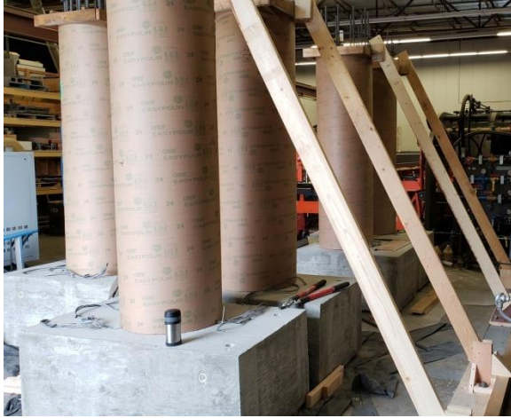
Figure 3.6: Construction: a) Bracing for Column Concrete Pour, and b) Bracing for Top Block Concrete Pour
