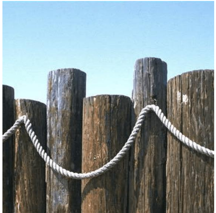
Figure 6. Wood used in docks and marine pilings should be treated to prevent damage by marine borers. Photo by: Gary Thomasson.
