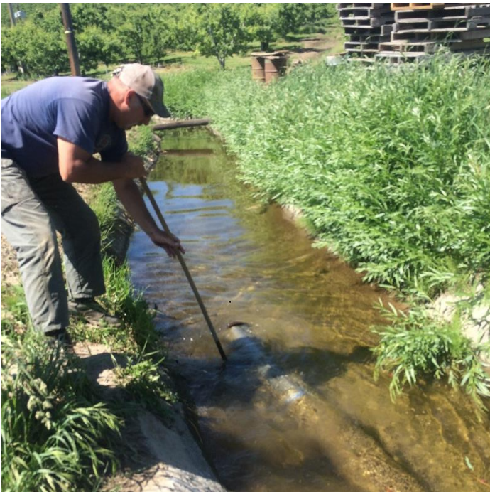
Figure 29. Grower cleaning irrigation canal filter.
