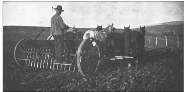
Fig. 9. An early model hoe grain drill with rows spaced eight inches apart. Seed was dropped through rotating flutes in the seed box down tubes behind the openers to the soil surface. Chains were attached behind each tube to lightly cover the seed with soil. Brumfield, 1968.
