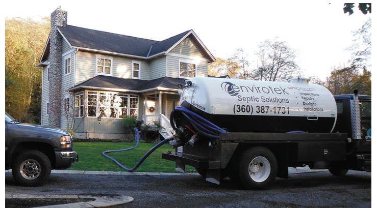
Figure 2. Pumping your septic tank is part of maintaining your system. Photo by Alan Chapin.
