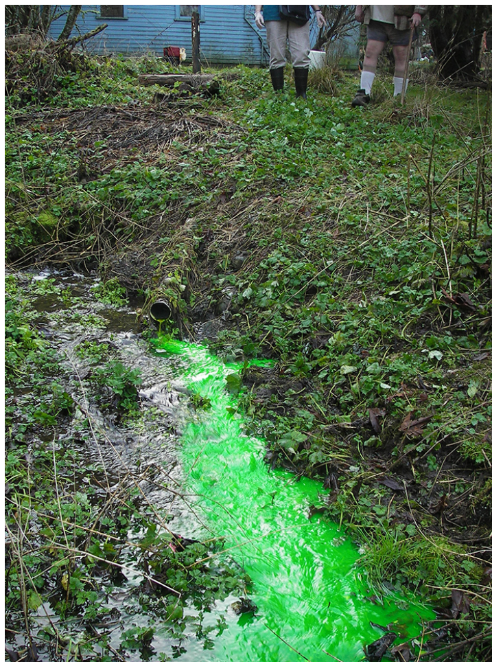
Figure 5. Dye test showing a failing septic system. Photo by Michael Dawson.
