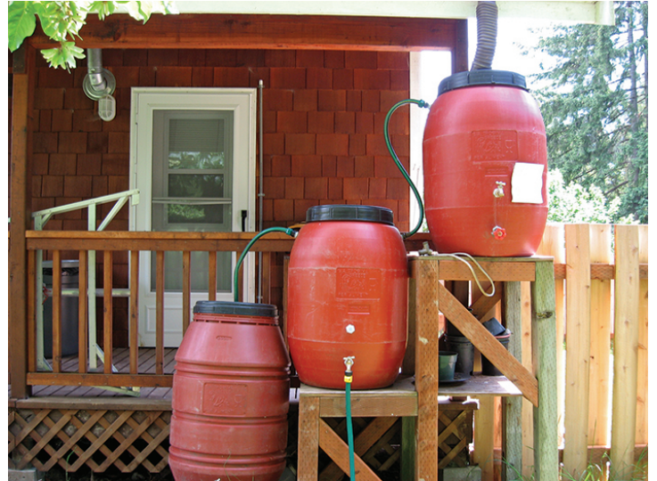
Figure 13. Rain barrels collect runoff that can be used later to water your landscape. Photo by Erica Guttman.
