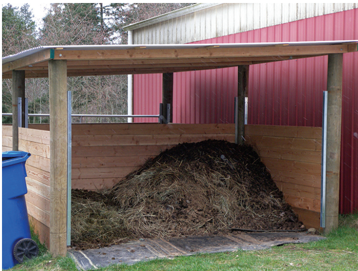
Figure 6. A properly covered manure storage area. Photo by Erin Ewald.
