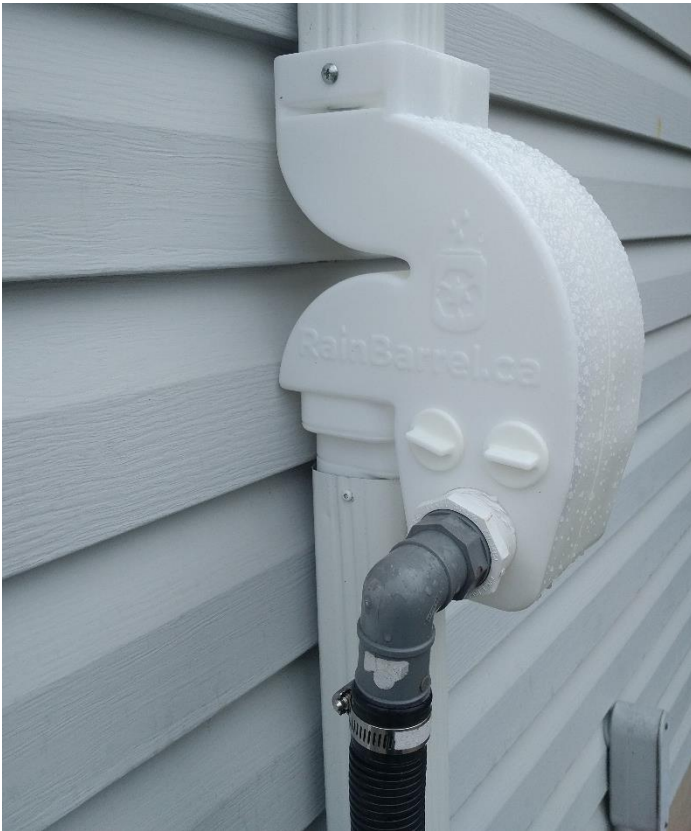
Figure 2. A diverter for protecting water quality in the barrel. Photo: M.J. Pilgrim.
