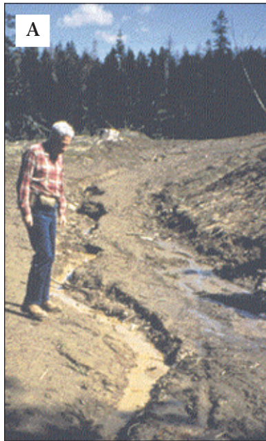
Figure 19. Unless guided into the forest to be filtered, erosion from forest roads can degrade adjoining stream water quality (A) and create small castle-like columns under gravel and rock. A 6-inch erosion depth suggests that as much as 50 cubic feet of soil could have been lost from a 100-square-foot area (B).
