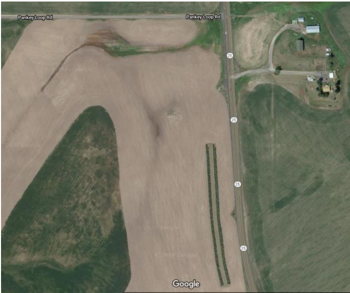
Figure 1. Davenport Living Snow Fence demonstration site, 14 miles north of Davenport, WA, on State Route 25, showing the twin rows parallel to the highway. This section of highway was selected based, in part, on WSDOT snow removal personnel recommendations. (Source: Google Maps.)
