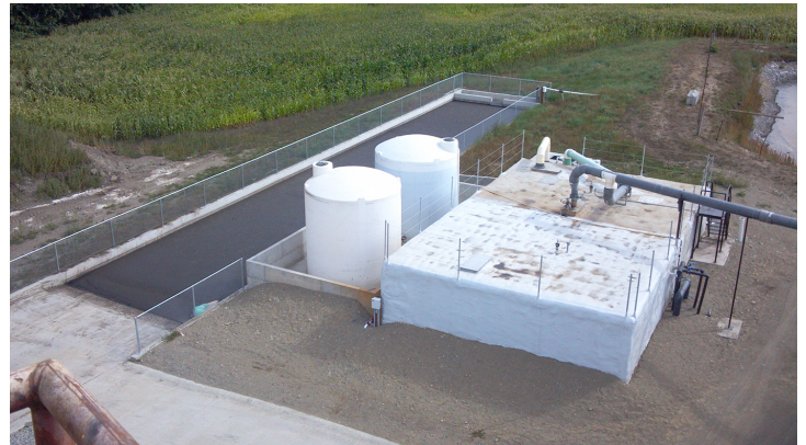
Figure 8. This nutrient recovery system, installed at a dairy anaerobic digester in Lynden, WA, produces ammonium sulfate, P-rich manure fines, and reduced-nutrient effluent. (Photo courtesy of Andgar Corporation.)
