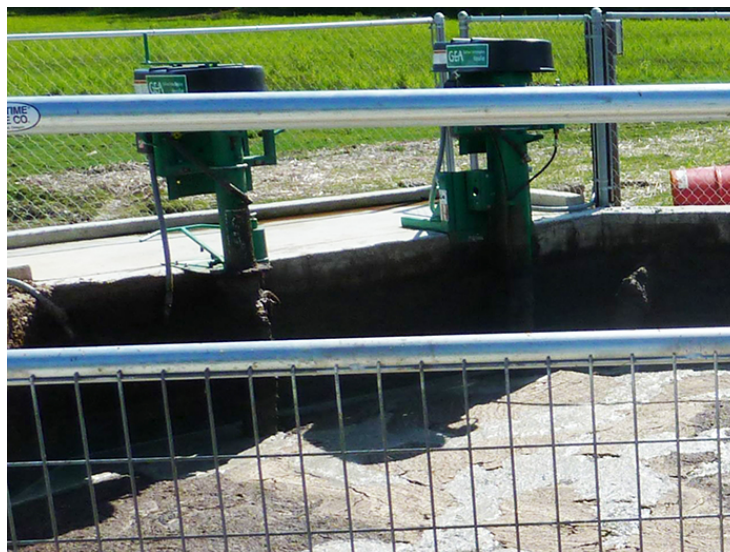
Figure 3. Mechanical mixers installed in this receiving pit homogenize the slurry (left), while an auger mixes food wastes with dairy manure (right). (Photos courtesy of Jim Jensen and WSU Energy Program.)
