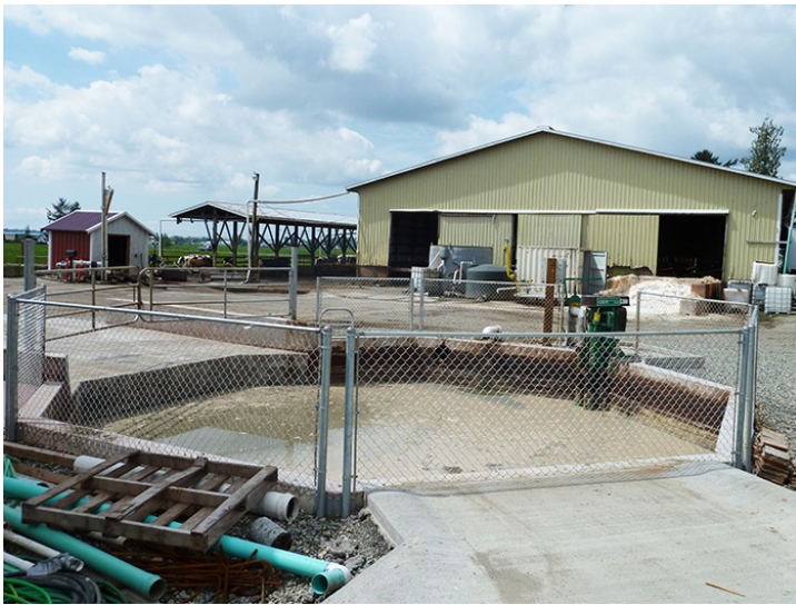
Figure 6. Added safety measures for waste haulers near receiving pits are another capital cost consideration associated with co-digestion. (Photo courtesy of Jim Jensen and WSU Energy Program.)
