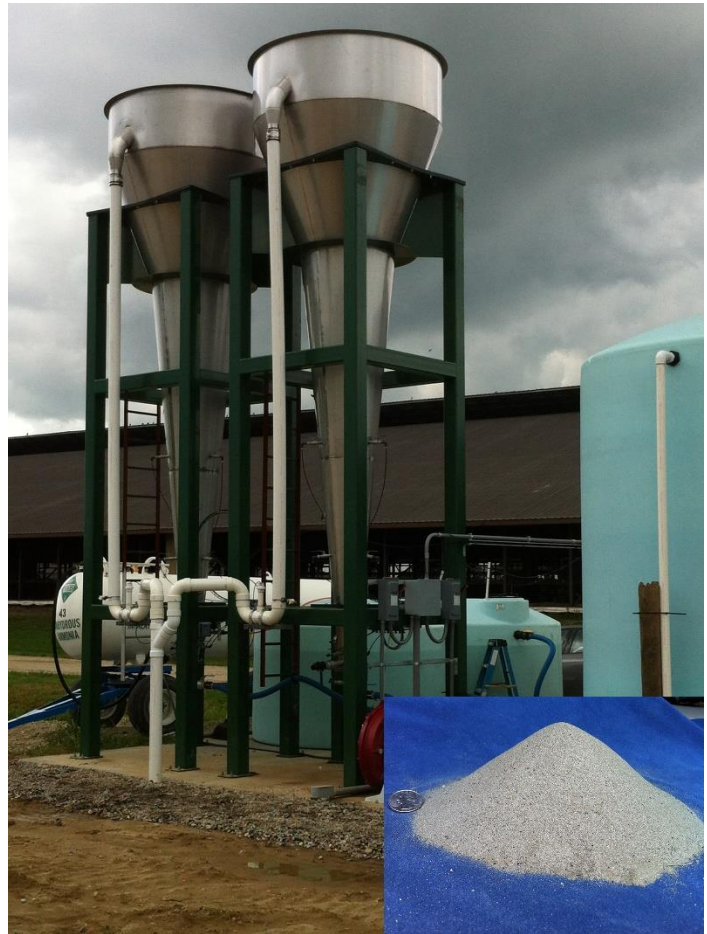
Figure 4. Struvite crystallizer and product (inset). Photos: MultiForm Harvest.
