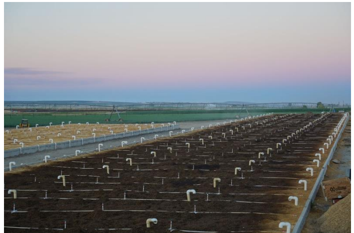
Figure 5. Vermifiltration system. Photo: Biofiltro.
