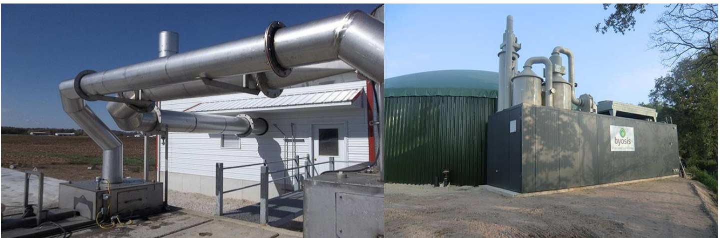
Figure 6. Non-chemical carbon dioxide and ammonia air stripper (left) and media tower ammonia air stripping (right). Left photo: DVO Incorporated; right photo: Byosis.
