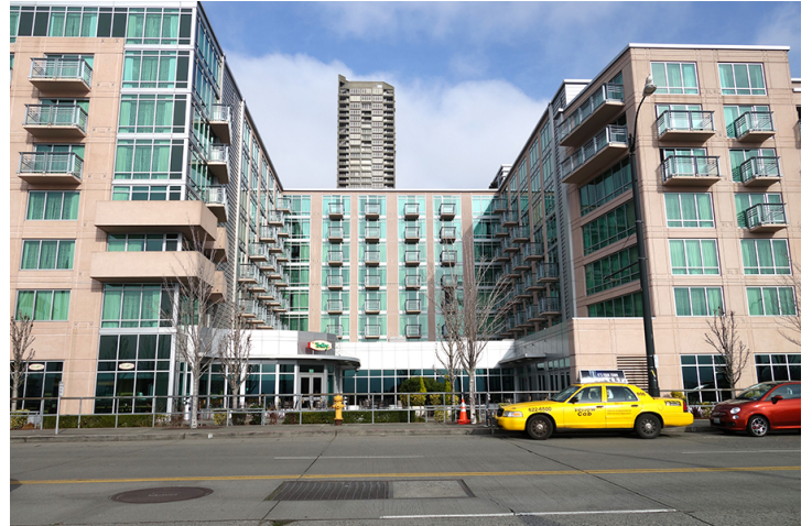
Figure 1. Deciduous trees have been planted on the south side of these urban apartment buildings in Seattle.
