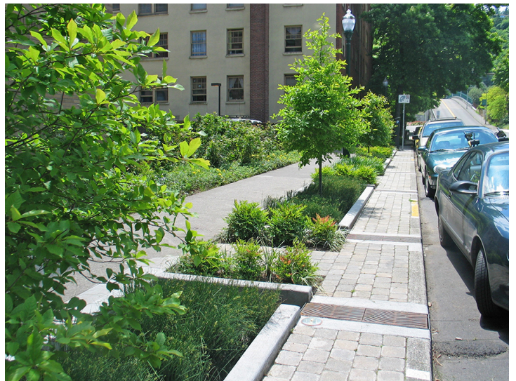
Figure 11. A stormwater street planter with green ash trees will filter the runoff from the street.
