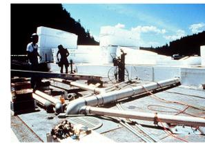
Fig. 3 - Drainage pipe layout during construction of the floating green
