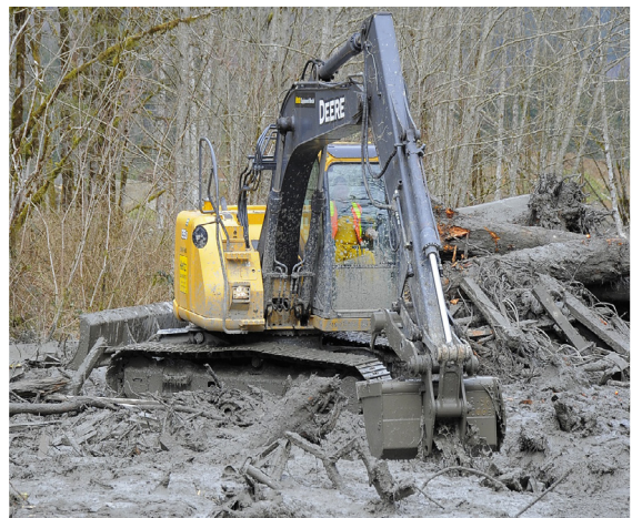
Photo: An Excavator Working in the Debris Field near Oso. Photo courtesy of WSP. Flickr/Snohomish County - CC: BY-NC-ND 2.0 https://www.flickr.com/photos/snoco/13455469653/in/set-72157642910921003
